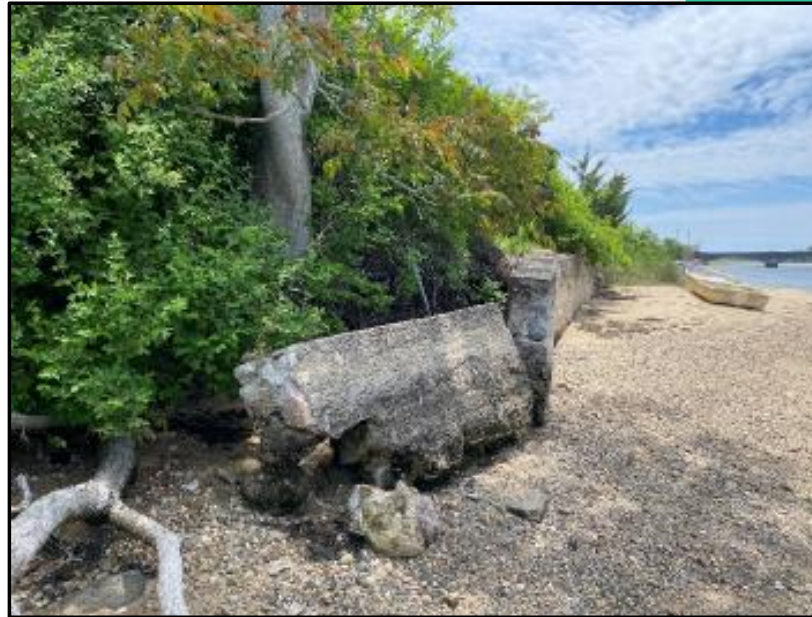
Photos 1, 2 – Deterioration of seawall and low-lying nature of adjacent municipal assets.
