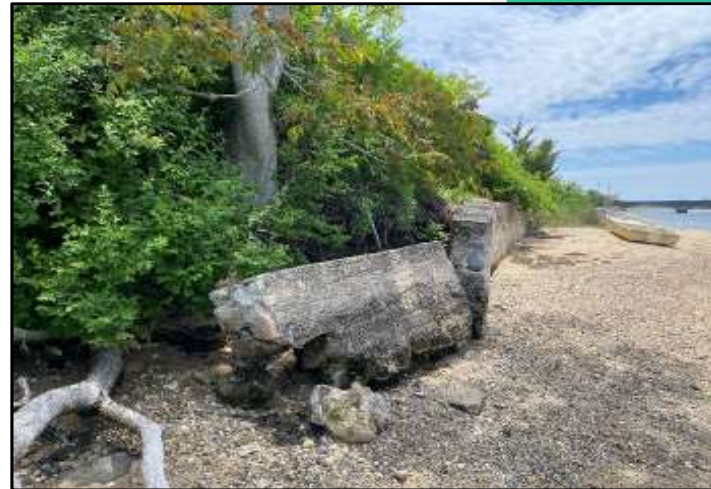
Photos 1, 2 – Deterioration of seawall and low-lying nature of adjacent municipal assets.
